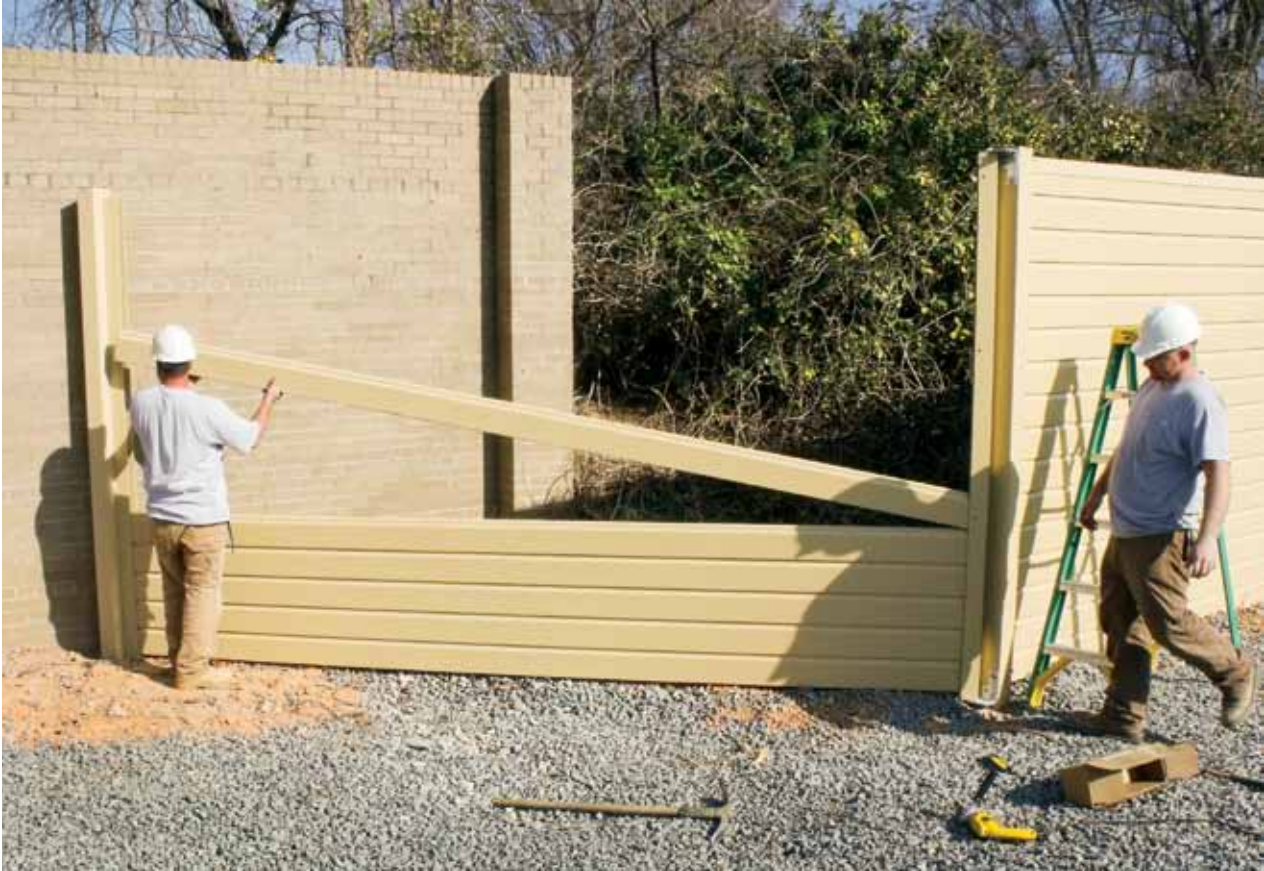
Carsonite sound barrier planks are adjustable and can be cut in the field.
