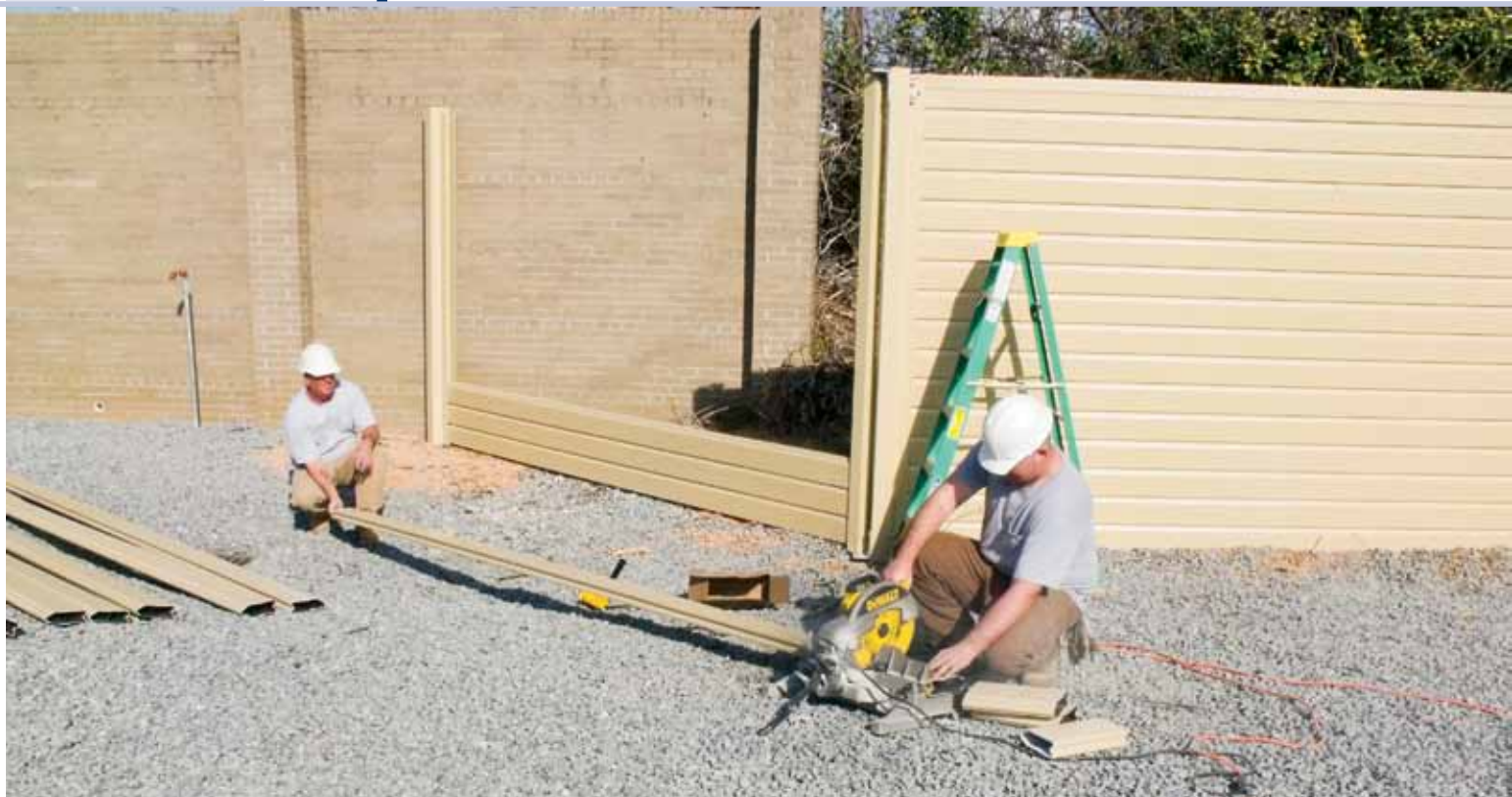
Carsonite sound barrier planks are adjustable and can be easily cut in the field.
