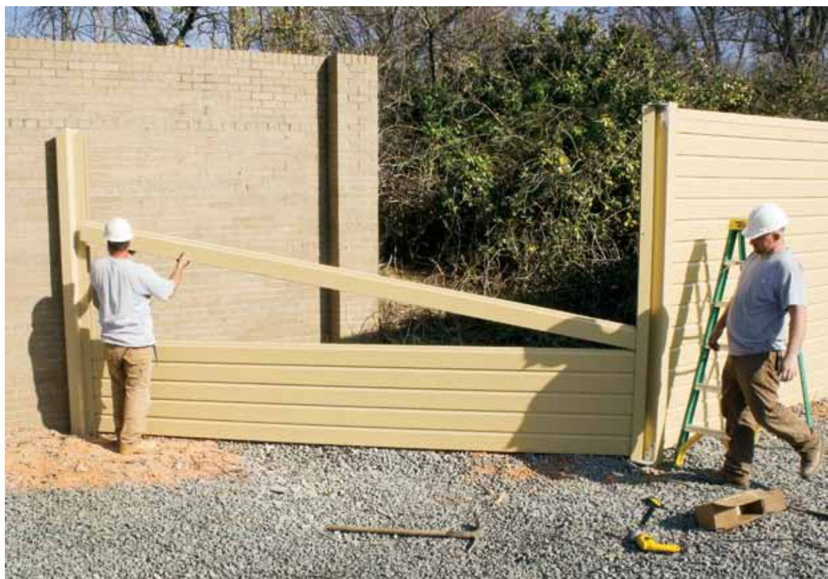
Carsonite sound barrier planks are adjustable and can be easily cut in the field.
